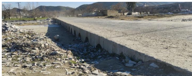
Figure 8. Pipes culvert before flood
